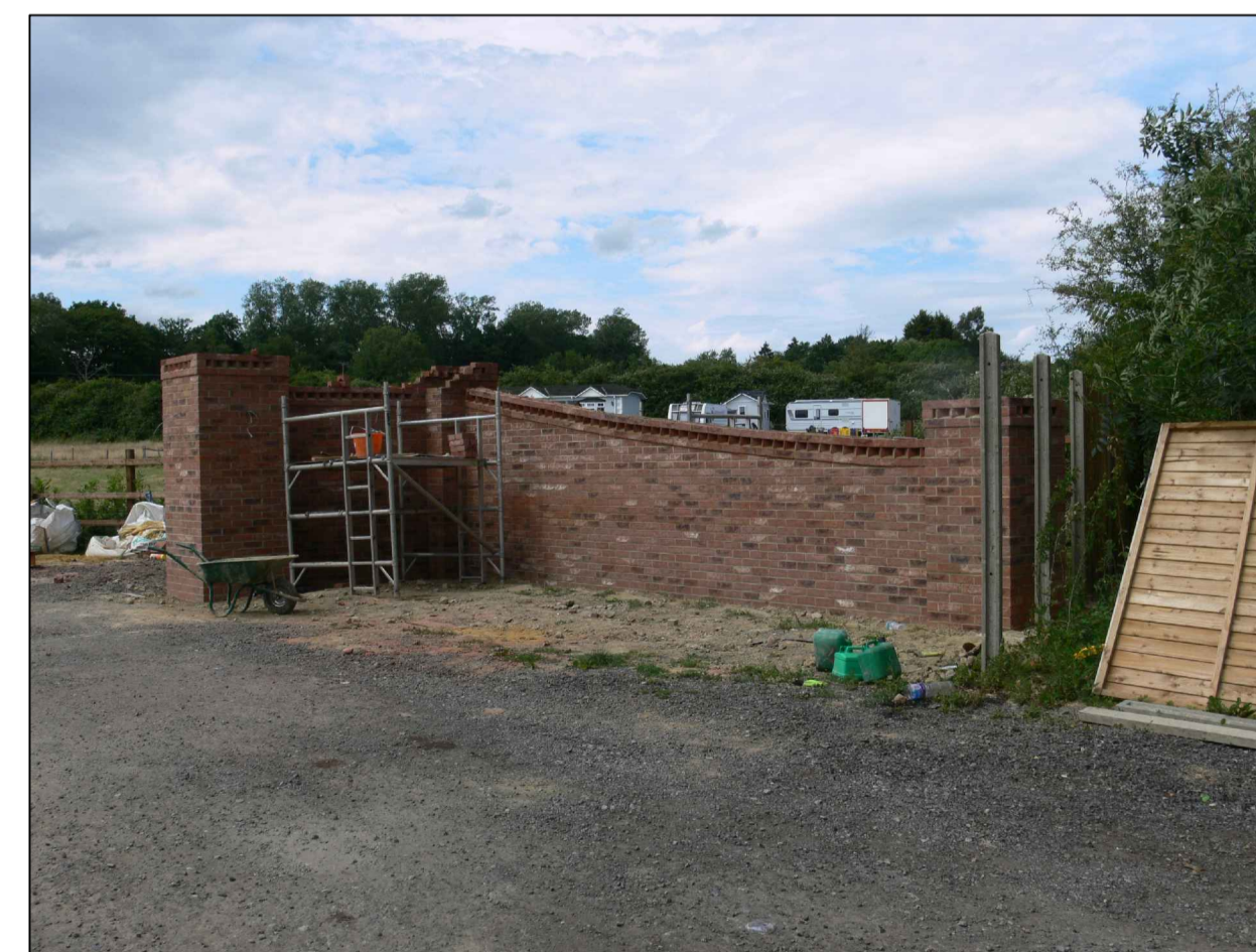
NOTE 3 - ENTRANCE WING WALLS
